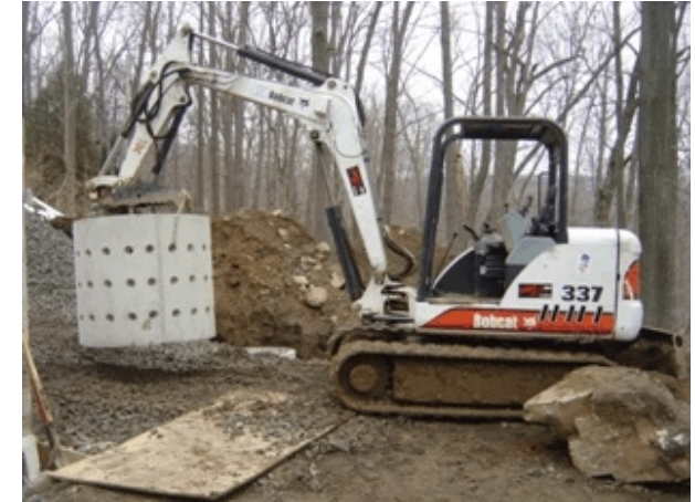
Typical Drywell Chamber - This tank is designed to allow water to flow out all sides and also the open bottom. Several feet of stone are placed below and around the tank as well.
