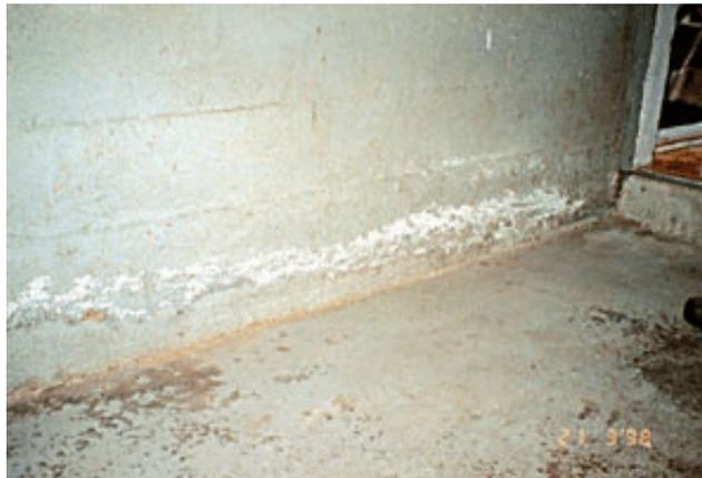
Efflorescence, a white powdery deposit found on the interior of foundation walls is usually caused by excessive moisture penetration through the wall. Efflorescence can usually be removed by scrubbing or chemical cleaning. If the condition
